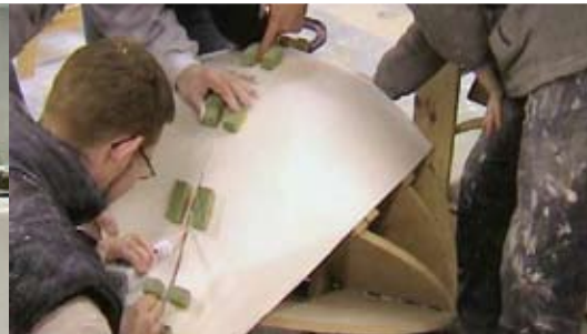
Applying DuPont™ Corian® joint adhesive to the seam
